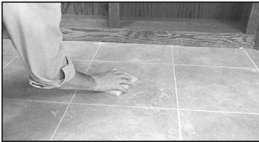
Fig. 30 - Use a 3M white, nylon pad to loosen grout residue.
