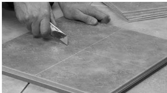
Fig. 3 - Score with a sharp utility knife.
