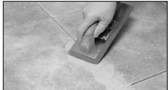
Fig. 28 - Pack the grout into the joints.
