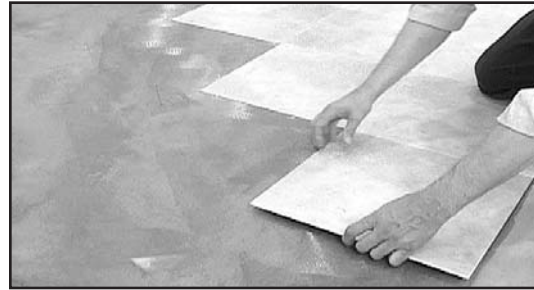
Fig. 15 - Install ungrouted floors following a stair-step pattern.
