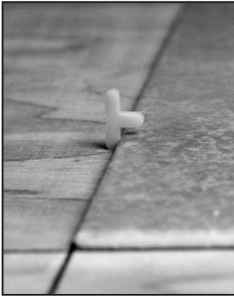
Fig. 12 - Use spacers with one leg removed.
